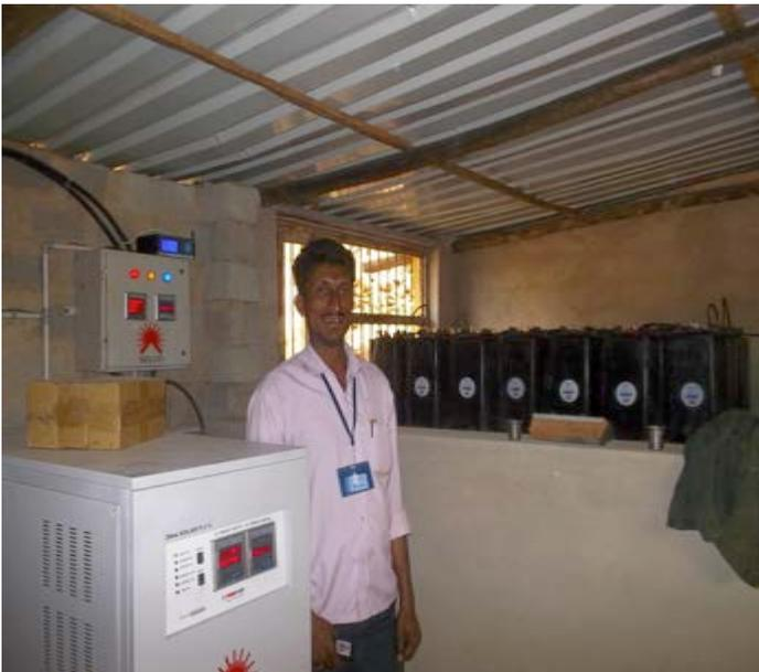
**20kVA Invertor, control panel and data logger system, Battery array in the background**
