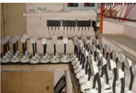
Solar lamps and charging station
