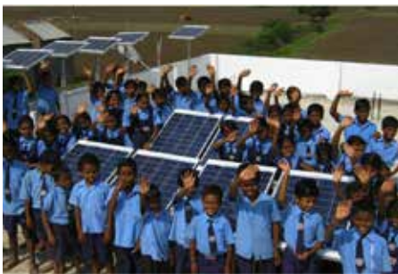
Solar Panels on the school terrace
