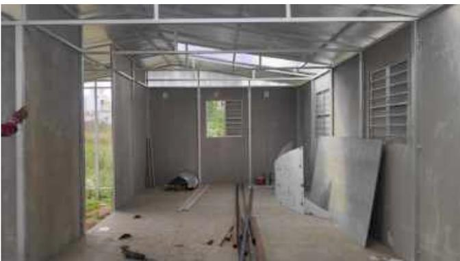
Due to long term leasing of the land, the structure built was also to be prefabricated, modular and portable to reduce wastage and reuse/rebuild with maximum of the construction material.
